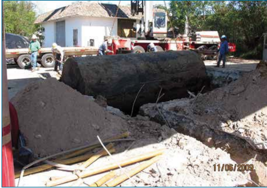
FIGURE 49. Leaking underground gasoline storage tanks are a common source of groundwater contamination.
